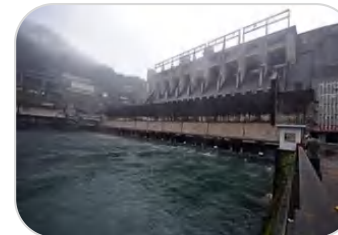
New anjiang Reservoir Dam
