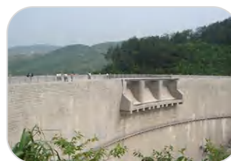
Shuangjiang Reservoir Dam.
