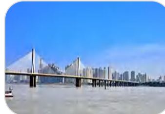
Xiangjiang River No2 Bridge
